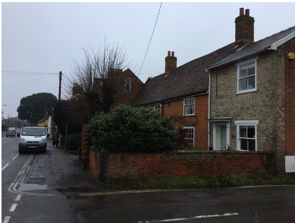
Figure 11 - Church Farmhouse and the adjacent 204 High Road.
