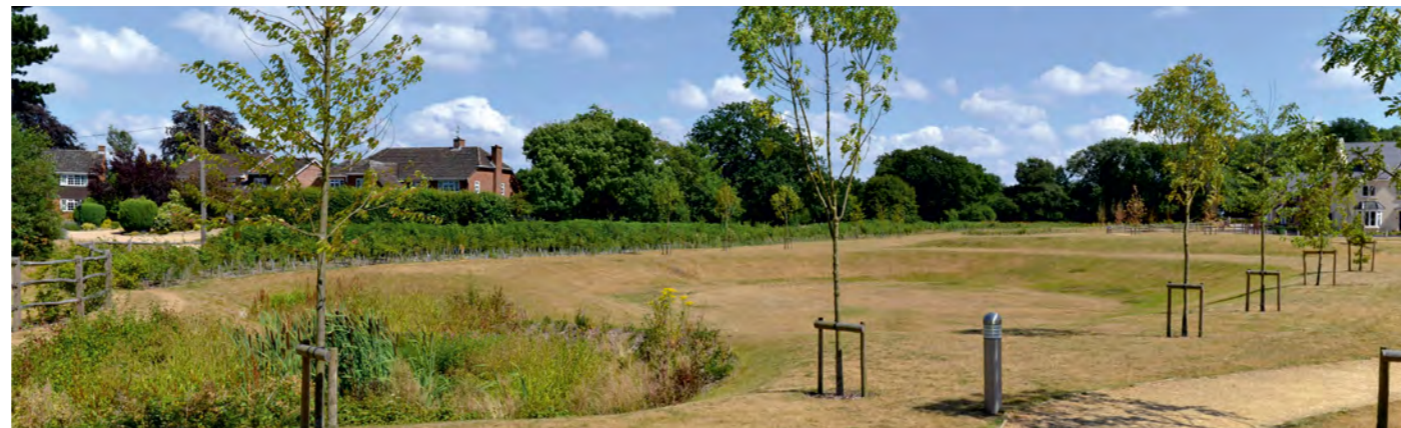
IMAGE 1: RETENTION POND THAT, IN DRY SEASON, CAN DOUBLE UP AS 'KICKABOUT' SPACE
